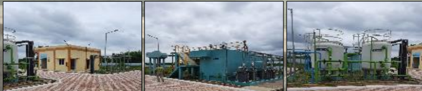
Storm Water Treatment Plant
